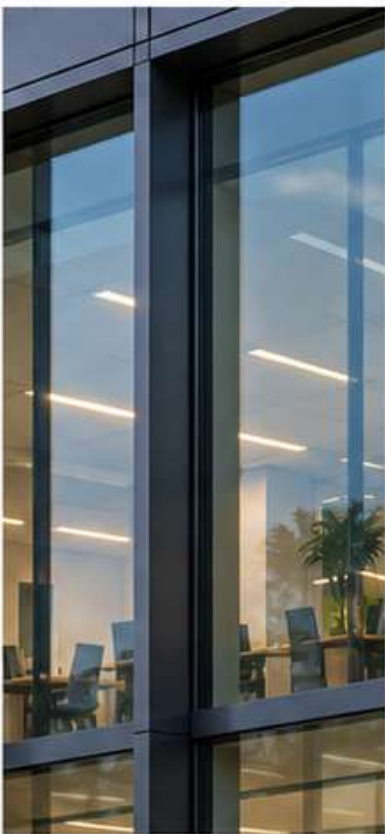
Recessed Glazed enclosure
